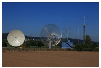
The antenna farm at HB9Q enables them to have great EME activity. It consists of a 15 m mesh dish for 144 and 432 MHz, a 10 m solid dish for 1296, 23xx, 3400, 5760, and 10xxx MHz, 8x19xxx M2 Yagis for 144 MHz, and 1x2.5wl M2 Yagi for 50 MHz, on top of the HF beam, 24 m above ground. (Photo by HB9CRQ)
