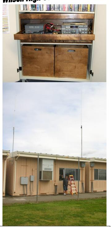
LBUSD Electronics Tech, Ray Barnum waves as the new Comet CHA-259BX vertical antenna installation is completed.
