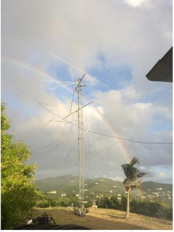
That's not a new antenna design, it's the aftermath of Hurricane Maria at NP2X. You can't see it here but even the tower has a broken base. Fred, K9VV, estimates wind speed at more than 200 mph. (Photo courtesy — Fred Kleber, K9VV)
