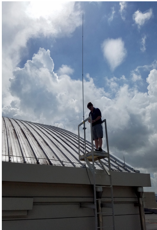
Volunteer Gary Sessums, KC5QCN, installs a VHF antenna on the roof of the Puerto Rico Convention Center. [Mike Corey, KI1U, photo]
