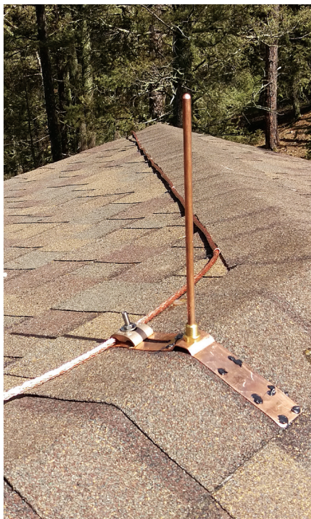
Figure 5 — Existing buildings can be retrofitted with lightning protection systems. [Photo courtesy of Mr. Lightning]
