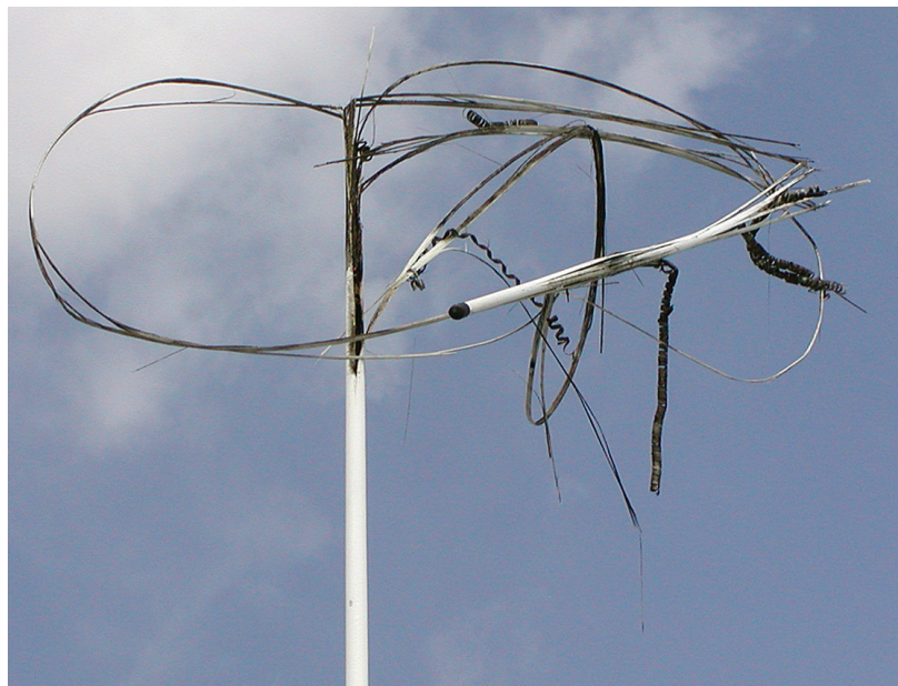
Figure 4 — Lightning destroyed this antenna. A properly designed and installed lightning protection system could have prevented this damage and provided protection for the owner’s home and its contents.
