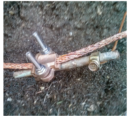
Figure 2 — The braided copper cable and large clamp are UL-listed for lightning protection and are much larger than the wire and clamp (near the top of the ½-inch-diameter grounding rod) required for ordinary household grounding. The two grounds are bonded to create a common ground point. [Photo courtesy of East Coast Lightning Equipment, Inc.]
