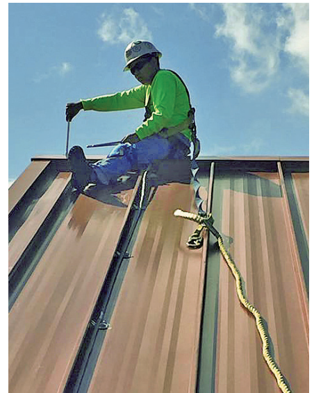
Figure 8 — Because much of a lightning protection system must be installed on rooftops or other high locations, it is advisable to have a trained professional with adequate protective gear do the work. [Photo courtesy of Labeled Lightning]
