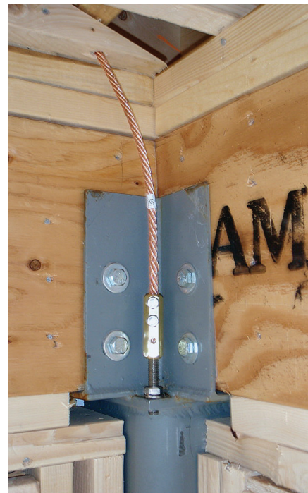
Figure 6 — A professional lightning protection installer can show you how to reduce the cost of an LPS. Here, for example, a conductor from the roof is connected to a steel column that acts as the conductor to the floor level and an external ground system. [Photo courtesy of Priestley Lightning Protection, LLC]
