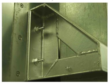
Figure 54 Welds on Galvanized Metal Supports
