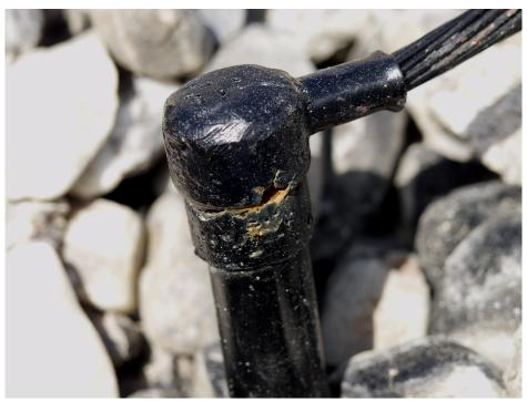
Figure 15 CADWELD<sup>®</sup> on Antenna Counterpoise Wire
