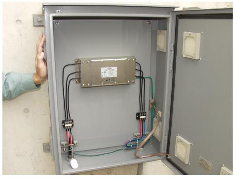
Figure 49 Improper Filter Configuration
