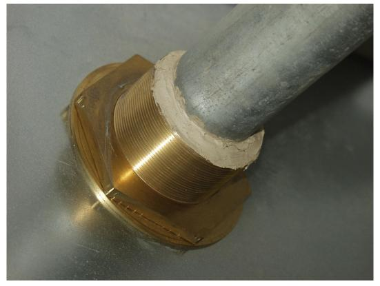
Figure 18 Water Pipe Penetrating a Shielded Room
