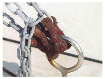
Figure 16 Example of a Rusty Joint
