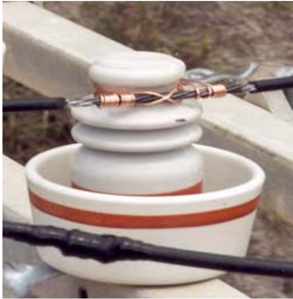
Figure 69 Tie Wire Source Mitigation, Example 2
