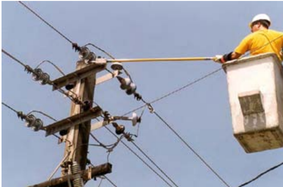
Figure 62 Source Identification with a Noise Sniffer
