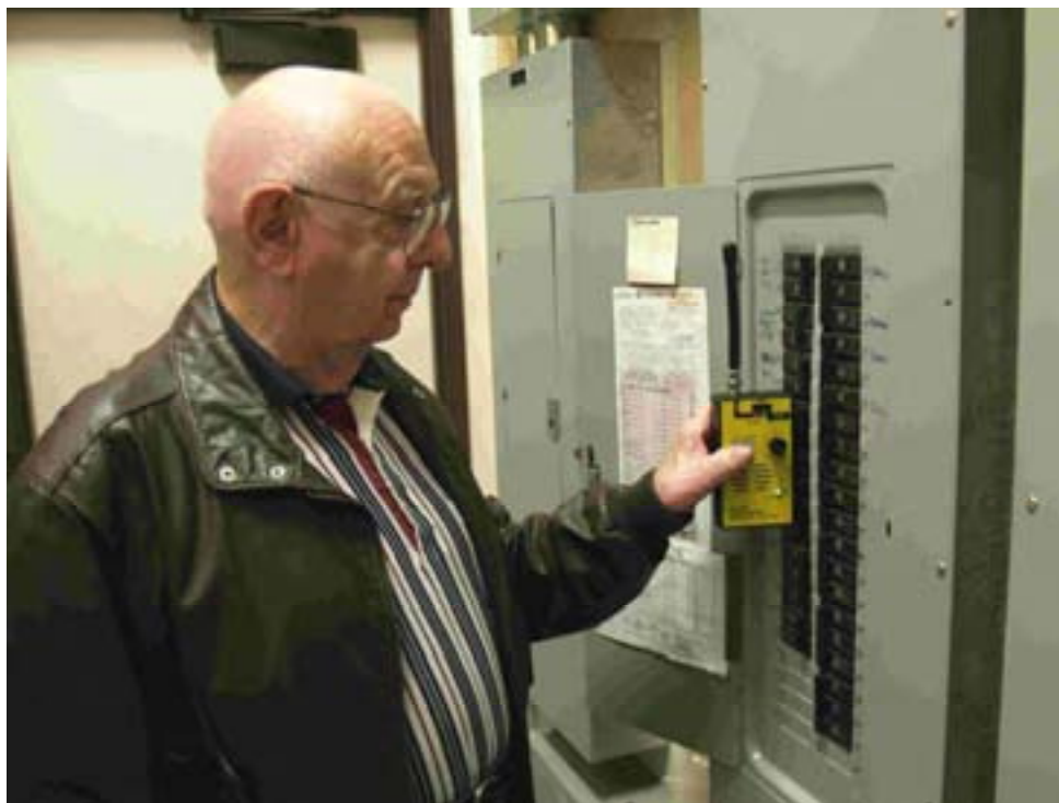
Figure 64 Using the Model 245 Circuit Sniffer
