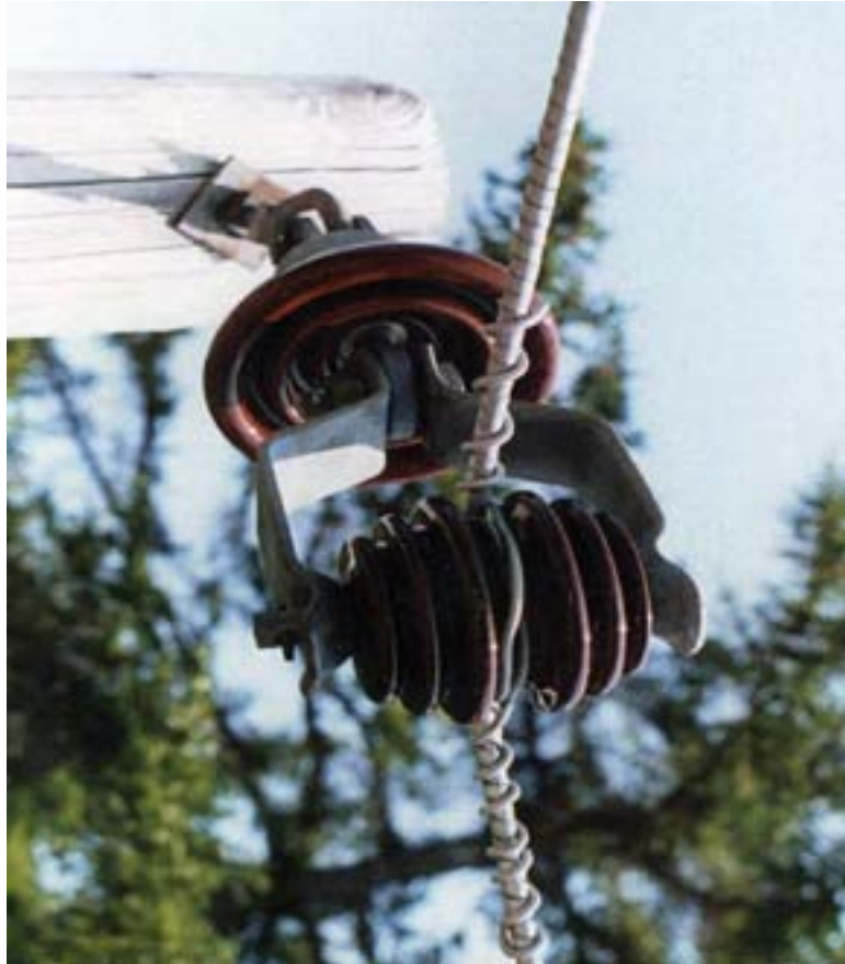
Figure 46 Spool with Insulated Tie Wire and Insulated Conductor
