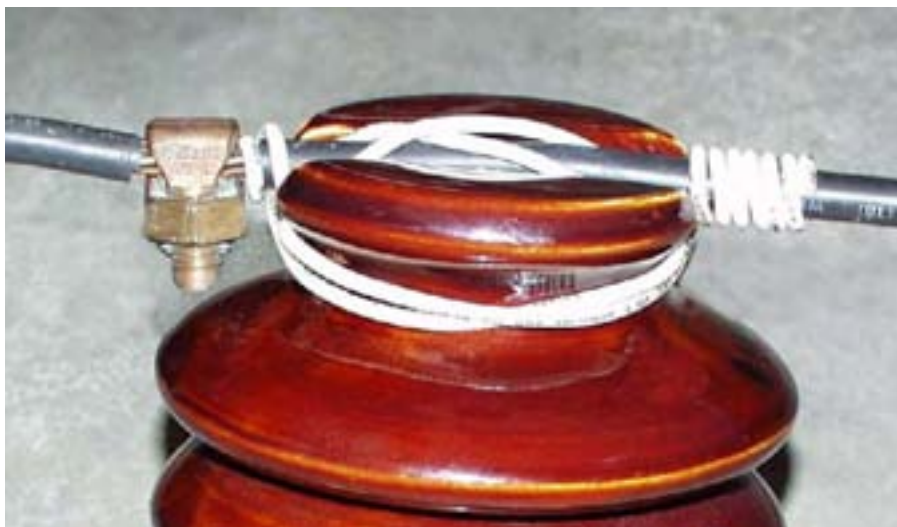
Figure 68 Tie Wire Source Mitigation, Example 1
